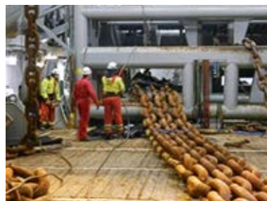
Installation. Spooling of the triple chain onto the anchor handling tug's work drum.
