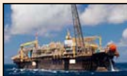
FPSO. Asset integrity management system in focus.
