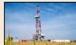
Gas production. Asset life extension.
