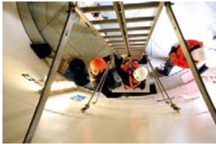
Training. EN 50308 requires that all parts of the turbine be accessible in a safe way.
