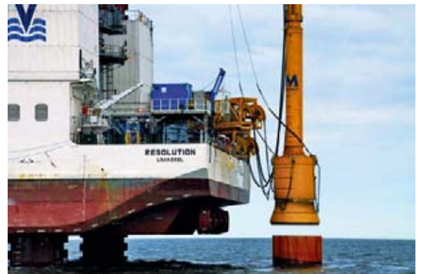
Ramming. Installation of a pile from a jack-up platform.
