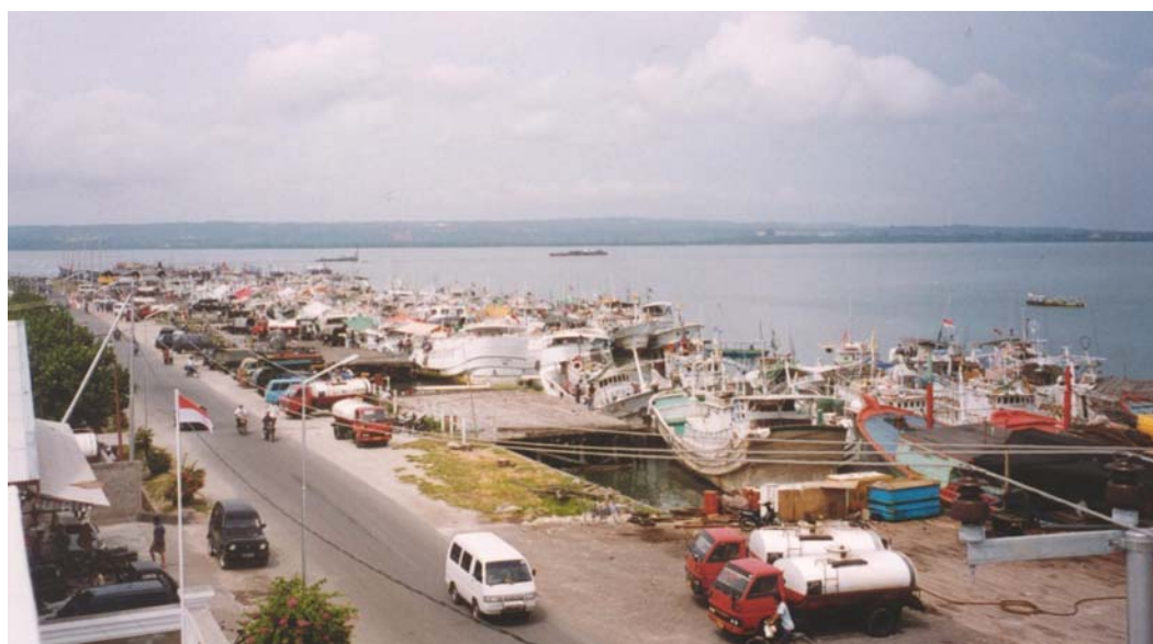
Figure 4.2.1. A section of the fishing vessel area of Port of Benoa.
