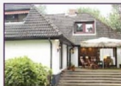
Walmdach-Bungalow Duvenstedt, KP 569.000 €
