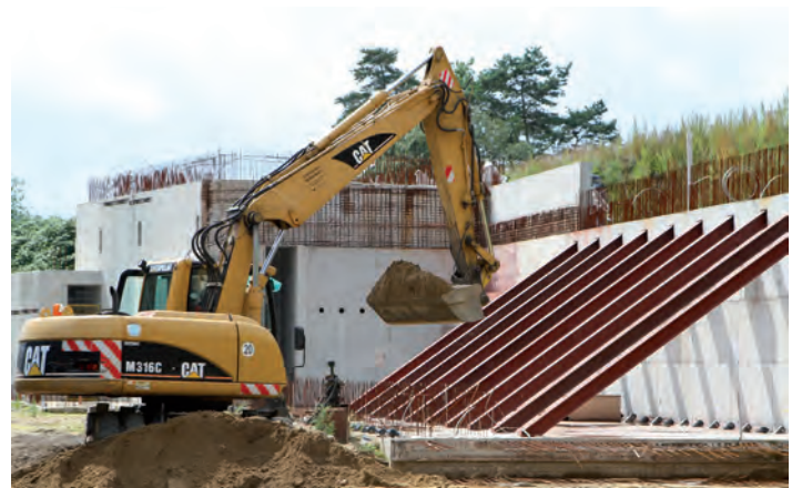
The FLASH II main tunnel starts to take shape.
