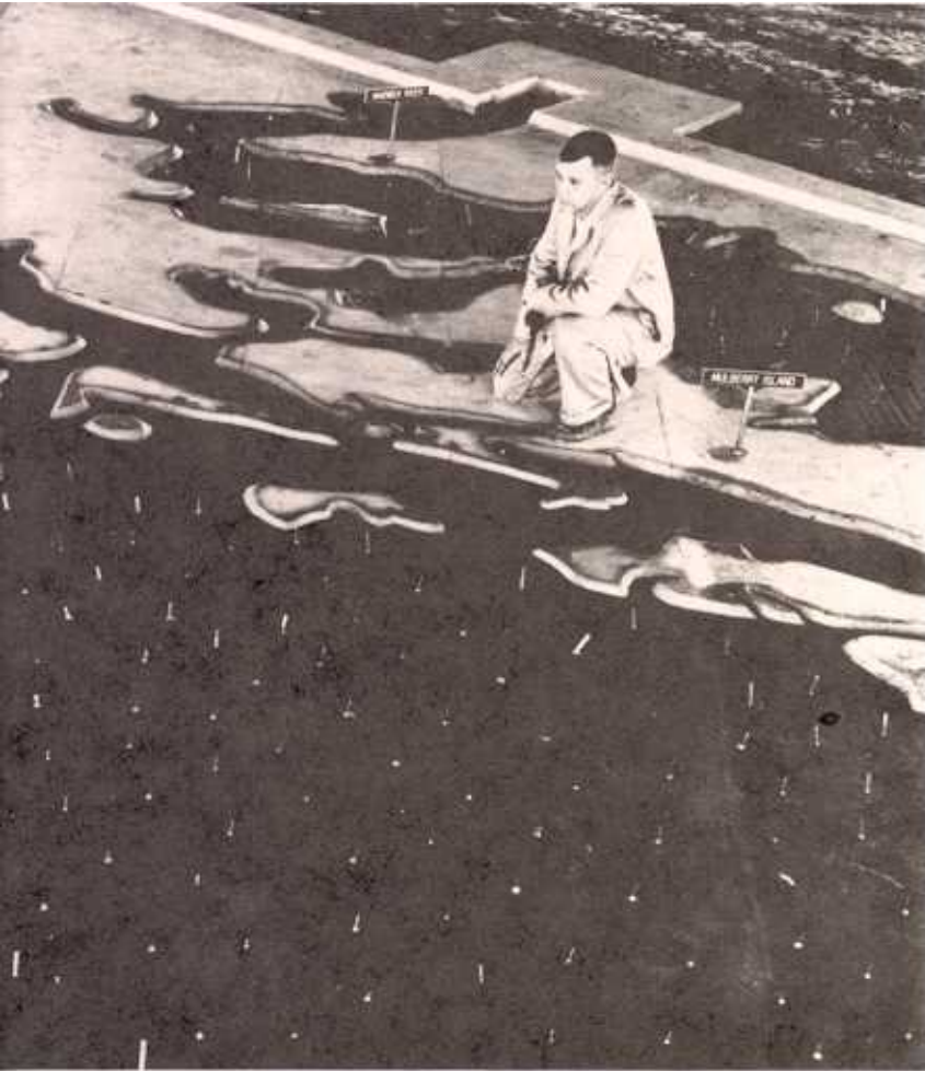
Portion of the James River model at the U.S. Army Engineer Waterways Experiment Station, Corps of Engineers, Vicksburg, Mississippi. This 1965 photograph shows the Rocklanding Shoal Channel. Salinities are reproduced to scale by operating the model with salt water in the downstream portions and introducing fresh water upstream to simulate upland runoff. (Courtesy Corps of Engineers)
