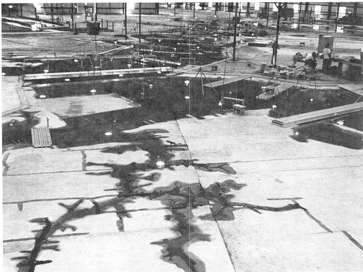
This photograph shows the James River Hydraulic Model. The catwalks allowed sampling for dye at points throughout the model, but required some gymnastic ability on the part of graduate students.
