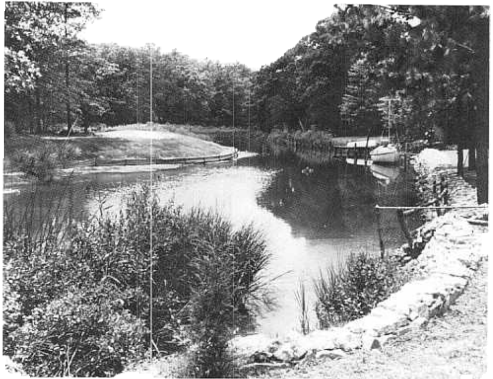
(above) This canal was widened by the Riverside Development Company to create a compensation marsh four times the original marsh destroyed by construction. A silt fence holds the newly-planted bank.
