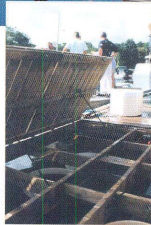
The upweller is built directly into the dock, allowing for ease of access and transport.
