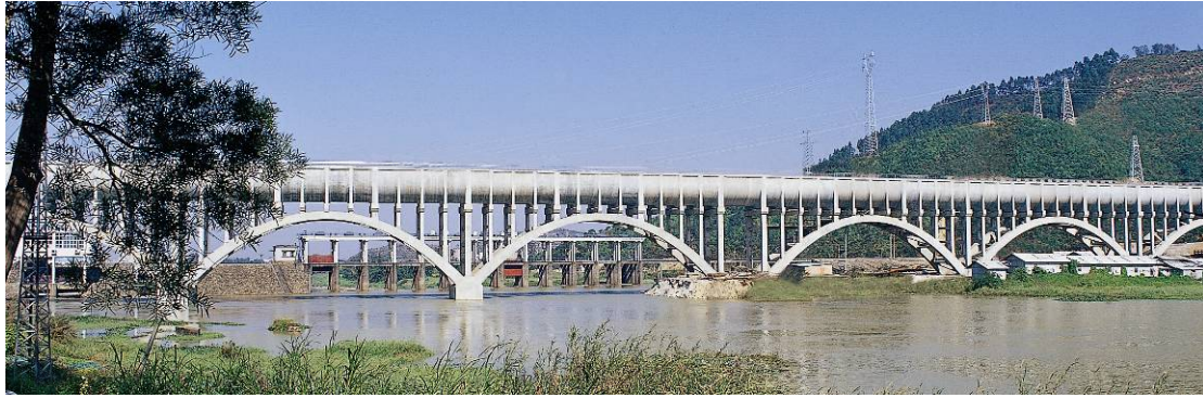
Fig. 7 Qiling aqueduct of Dongjiang–Shenzhen water supply project
