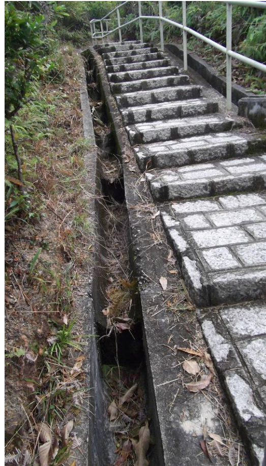
Fig. 9 Rainwater collecting channel at hillside
