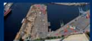
Buss Ross Terminal
