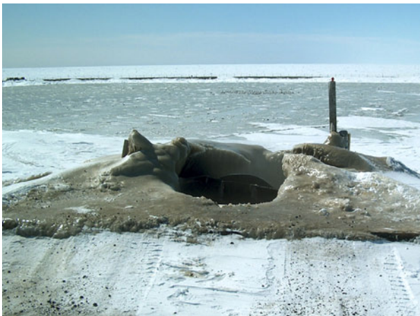
Sewage disposal site , Arviat, Nunavut
