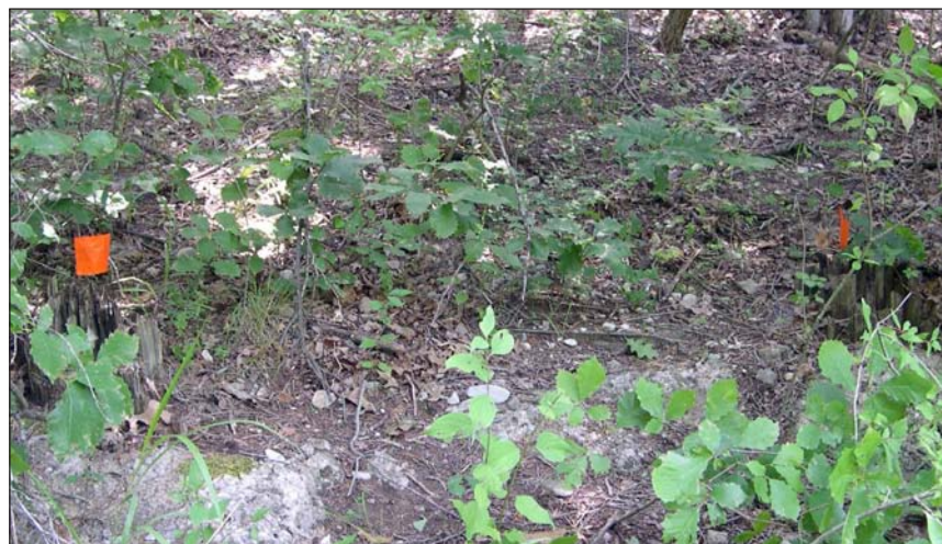
Figure 15. Conglomerate and concrete footing and wood post remnants (flagged) of historic sign at Antelope Spring.
