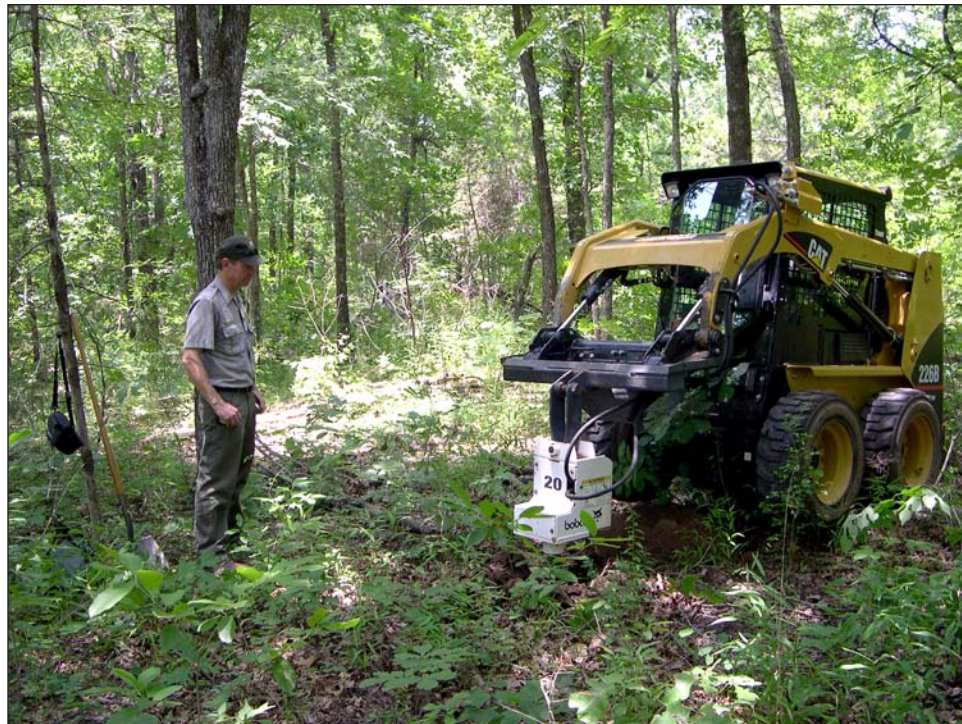
Figure 9 . Conducting auger tests near Buffalo Springs Comfort Station.
