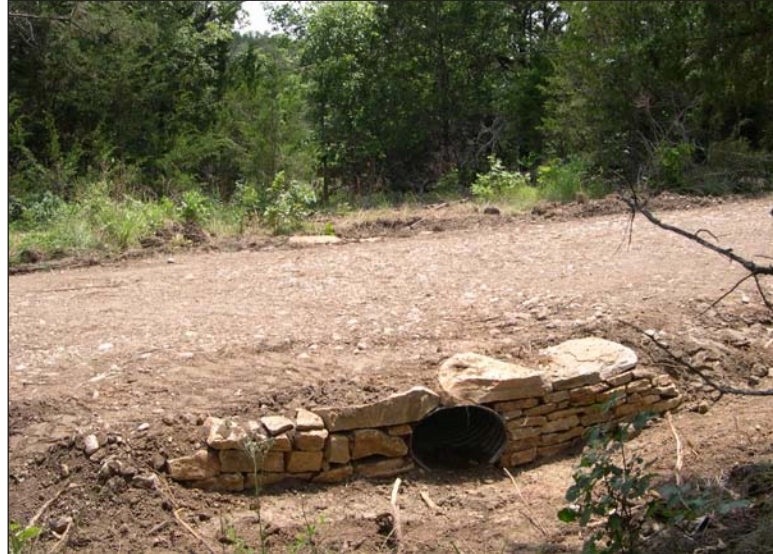
Figure 6. Example of gravel road rehabilitation associated with Culvert “M” looking south.
