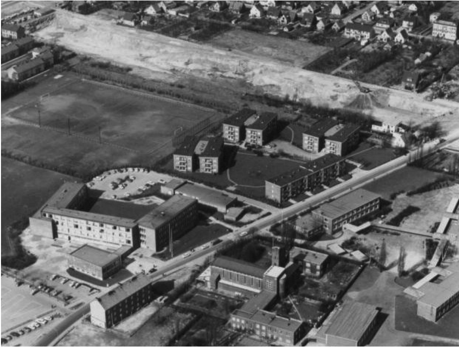
U-Bahn-Bau in Billstedt
