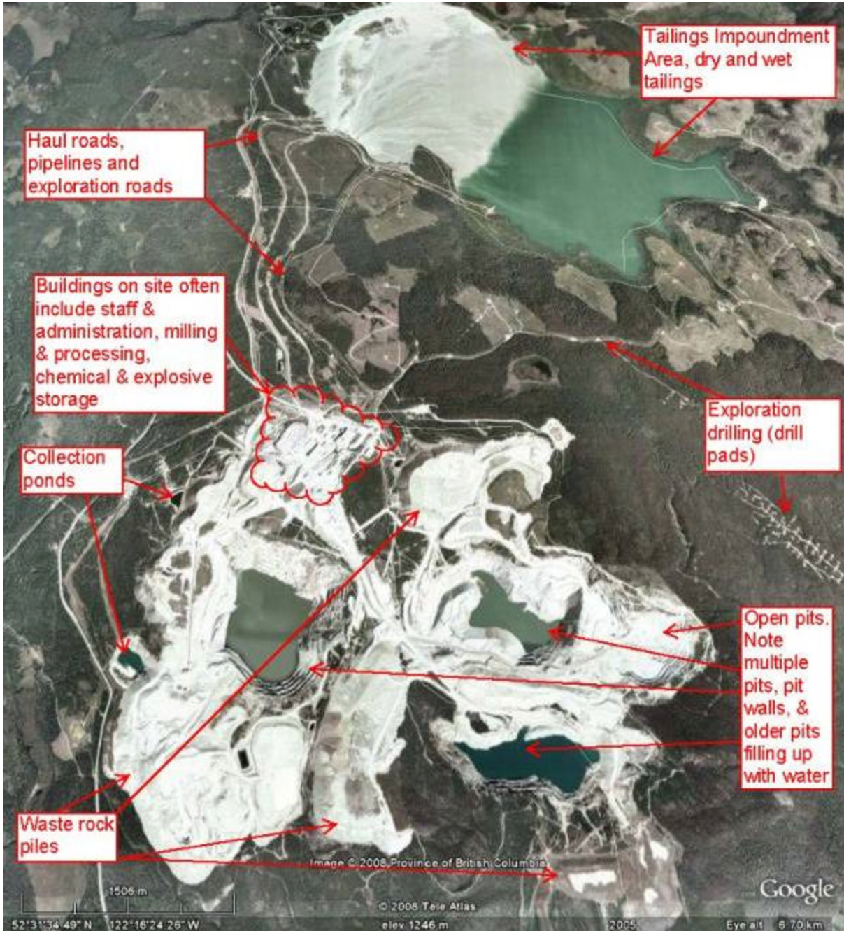
Although every mine is different, here is an example of some common mine site components. (Photo: Gibraltar Mine, BC. GoogleEarth, July 2008)
