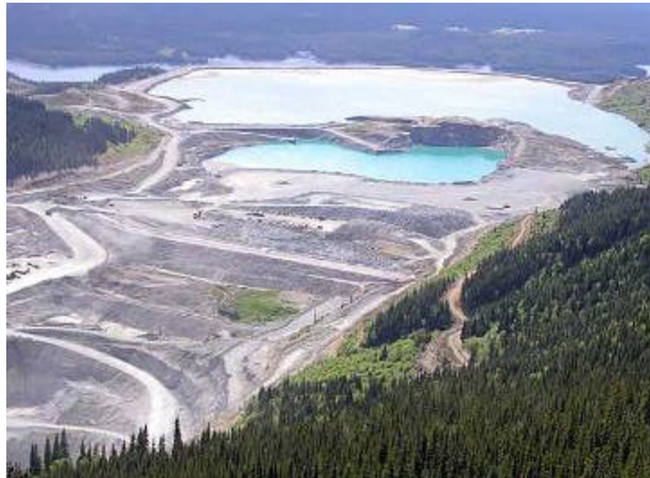
From background to foreground, Tahtsa Reach, tailings impoundment area, flooded pit, open pit at Huckleberry Mine, BC. http://www.bcminerals.ca/files/bc_mine_information/000089.php
