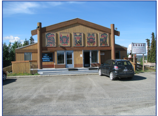
Teslin Tlingit Council Administration Building, Teslin, Yukon
