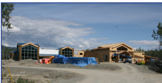
Dä Kų Cultural Centre under construction, July 2011
