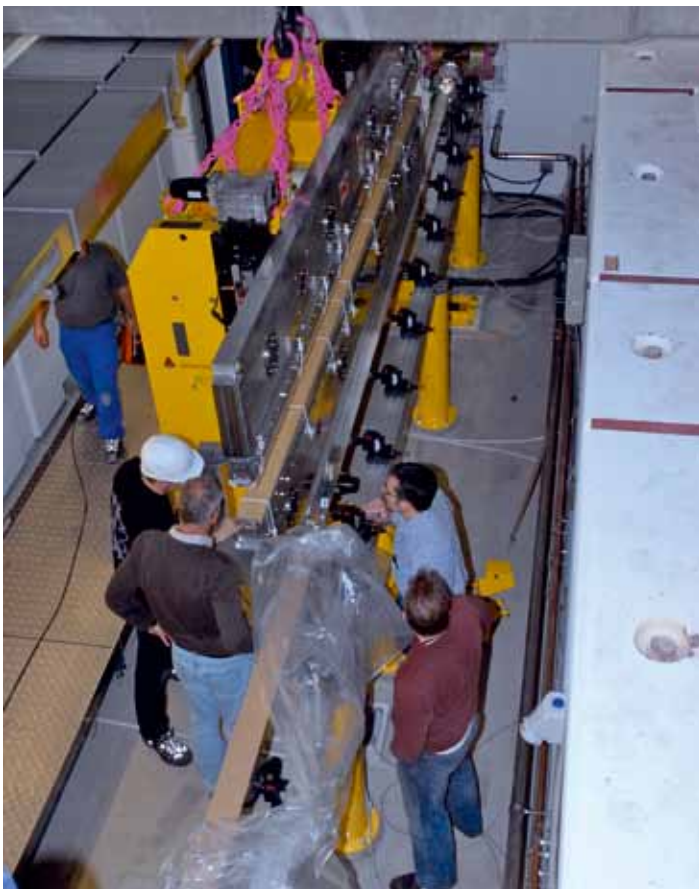
Figure 2 The first 5 m undulator module being installed at beamline P01 (November 2010).
