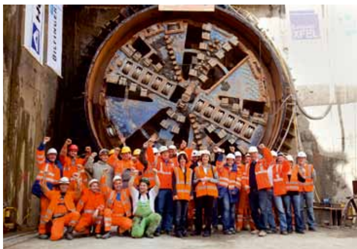
The tunnel builders with the two patronesses (left: Imke Gembalies, right: State Minister Dr. Herlind Gundelach) in front of the cutterhead of TULA. The rest of the borer is still located inside the newly completed tunnel section.
