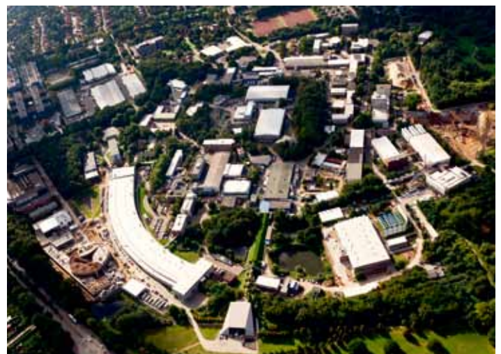
An aerial view of DESY with the photon sources PETRA III, FLASH, and DORIS III. The construction site of the new CFEL building is on the left side of the curved PETRA III experimental hall (September 2010).
