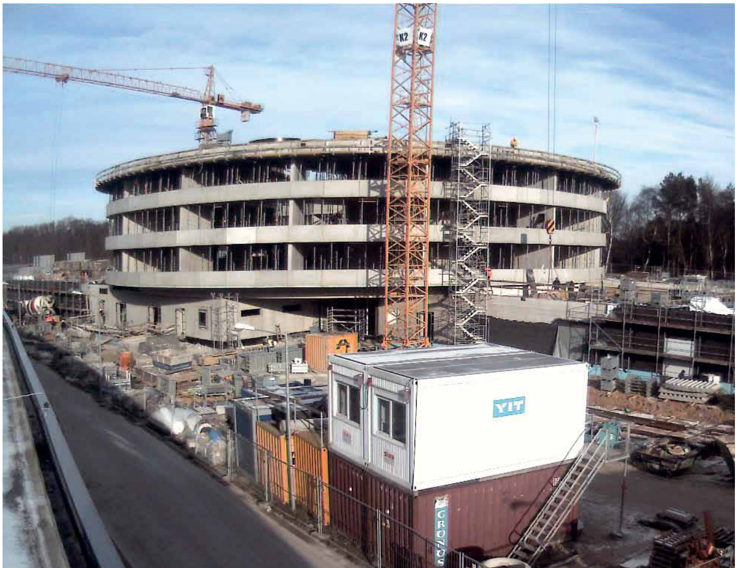
Figure 2 CFEL construction site on 1 December 2010.
