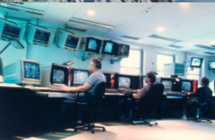
In the control room of the HERA refrigeration plant
