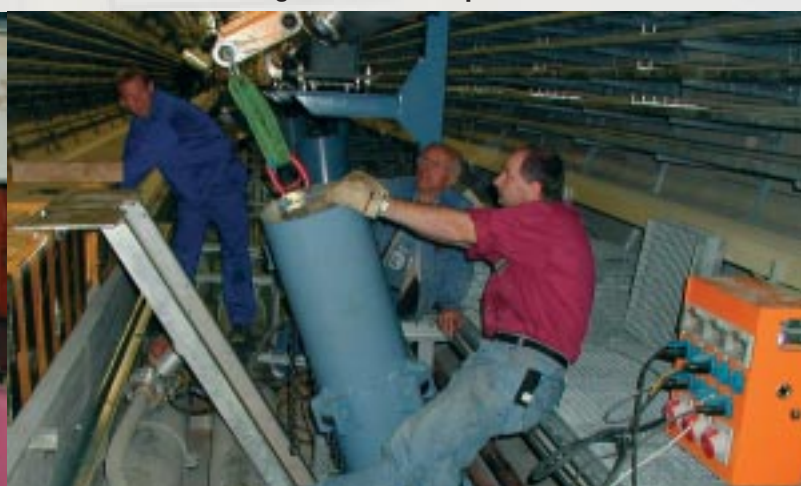
Assembling the spin rotator supports: This section of the accelerator can be raised and lowered as though it were on a platform lift.
