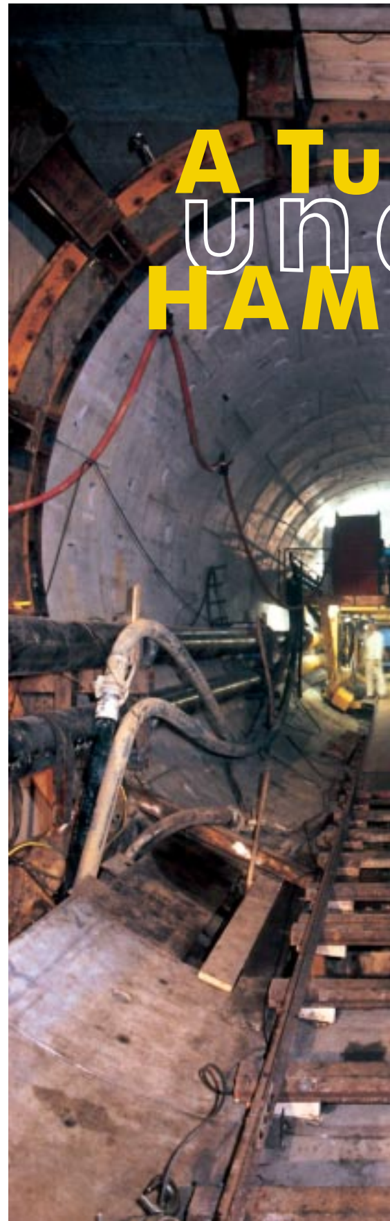
Light at the end of tunnel: Work on the HERA ring advances; the boring machine HERAKLES can be seen in the background.
