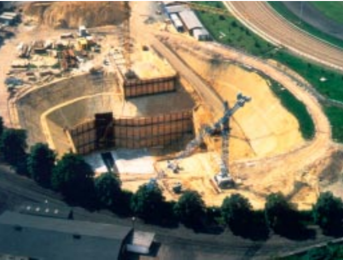
The four underground HERA halls were constructed by open excavation.
