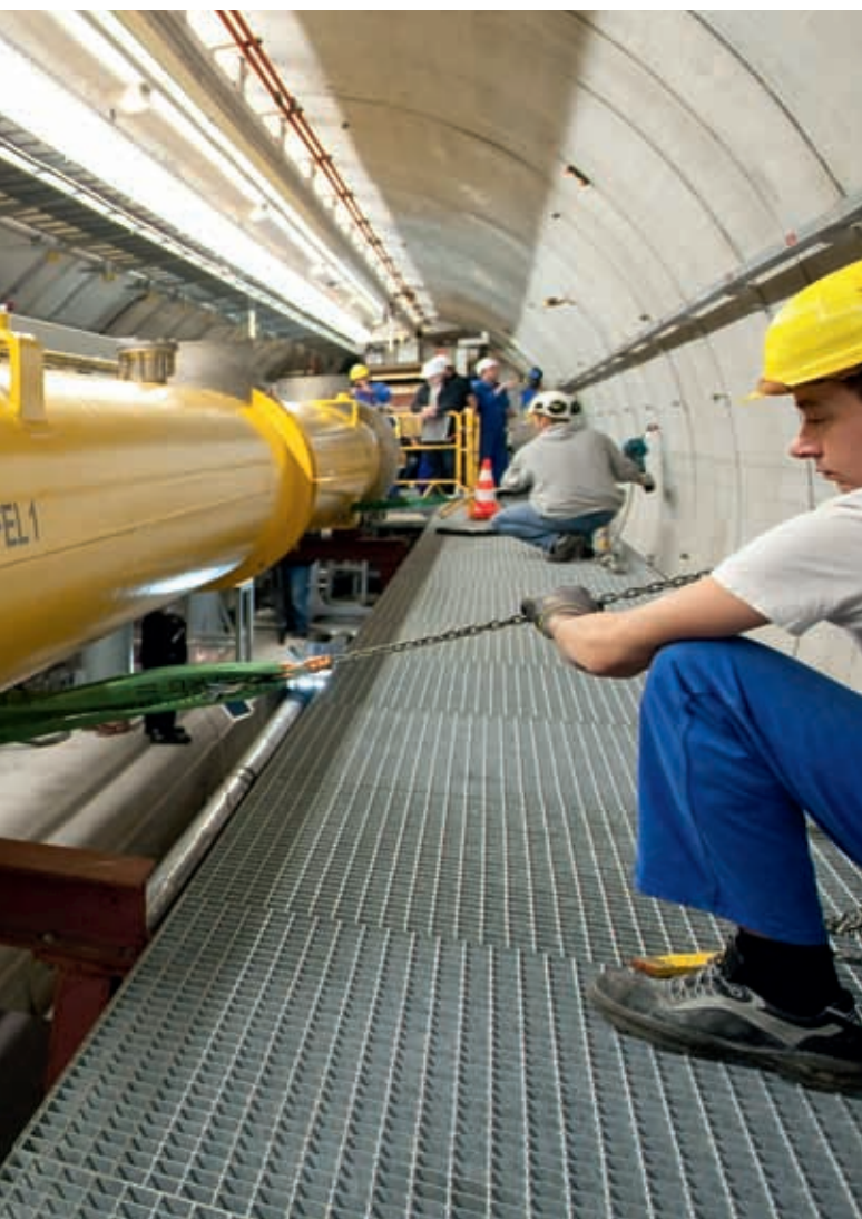
● Installation of a superconducting accelerator module in the free-electron laser FLASH
