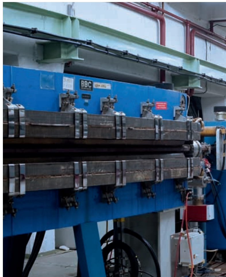
Inside the DORIS accelerator tunnel
