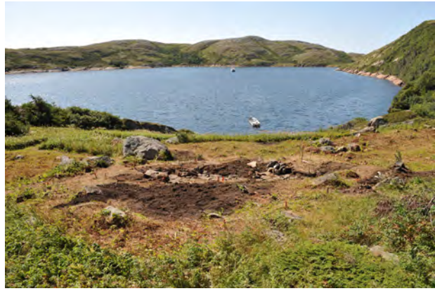
Fig. 5.09: Site backfilled. Photo by Wilfred Richard.
