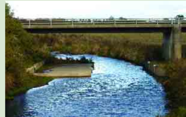
The River Nidd at Skip Bridge. By replacing a gauging weir with an ultrasonic flow gauge, a major obstacle to fish migration has been removed. This has led to an upturn in angler catches.
