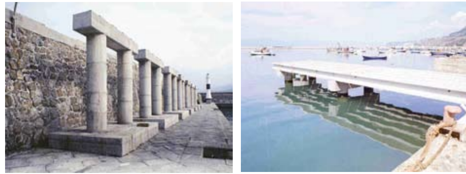
FIGURE 20 Precast concrete trestles (left) and concrete jetty under construction (right)
