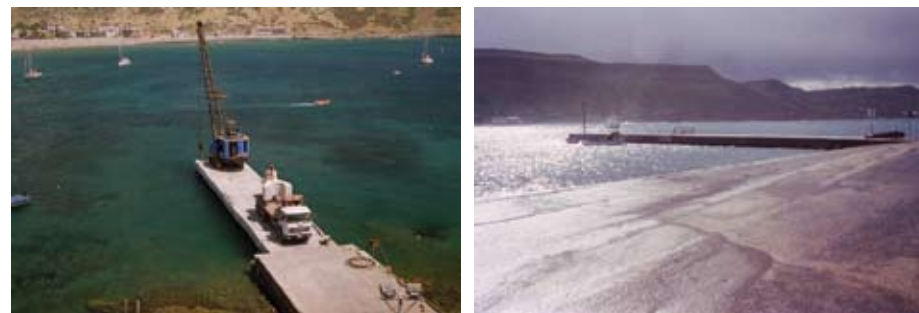
FIGURE 22 Concrete jetty built with modular units from land
