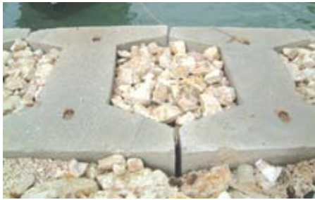
FIGURE 28 "I" blocks in-filled with rock
