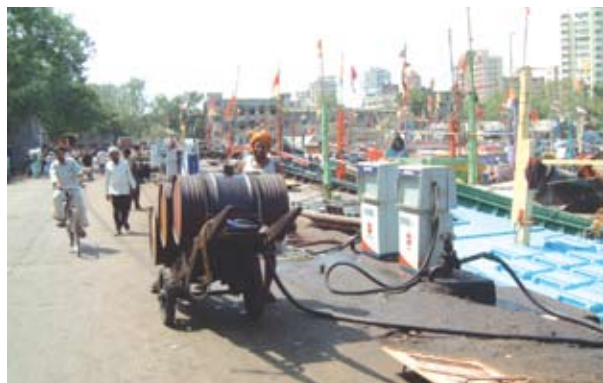
FIGURE 24 Unsuitable fuel pumps for trawlers (flow rate 40 litres/minute)
