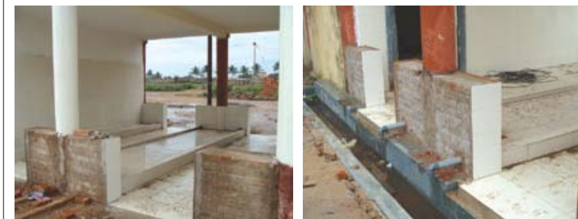
FIGURE 31 Crouching-only sorting platforms under construction
