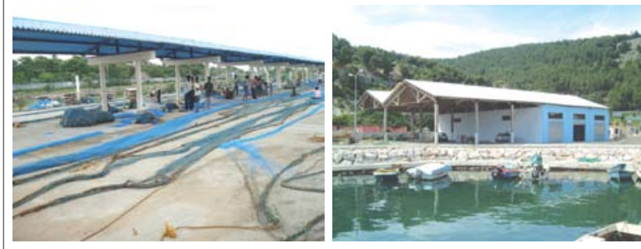
FIGURE 43 Large-scale net repair structures
