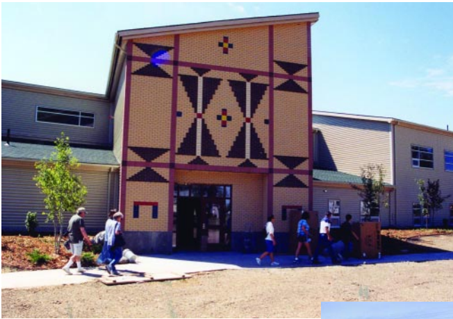
Academic building entrance
