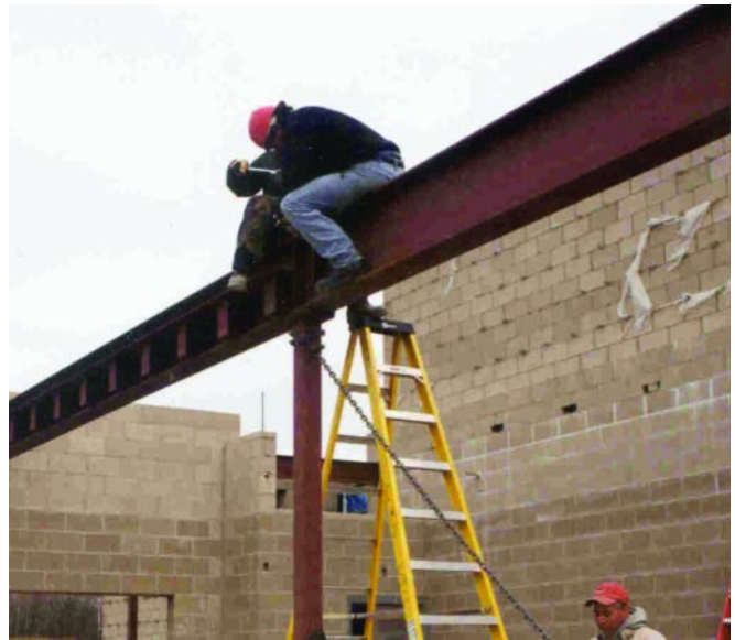
Performing arts center under construction
