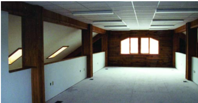
Upper level of the cultural learning center
