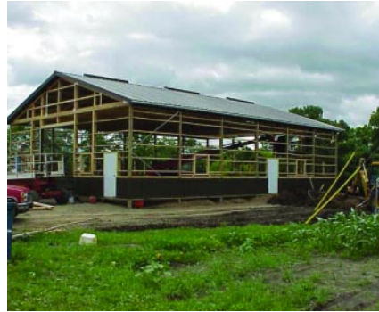
Vocational building under construction
