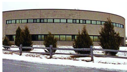
Piya Wiconi Bldg
