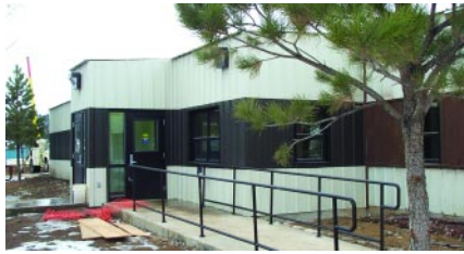
HVAC system and ADA ramp additions
