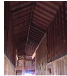
Academic building under construction
