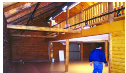
Interior of cultural learning center
