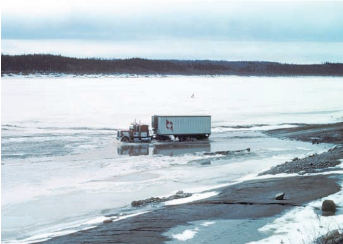
FIGURE 17: Transport truck crossing deteriorating ice road, Liard Ferry crossing near Fort Simpson, Liard River, NT (Terry D. Prowse).
