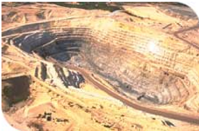
Figure 3. Deilmann open pit at Key Lake mine, in 1994. In 1996, the pit was converted to a tailings management facility and now receives tailings from the McArthur River mine.
