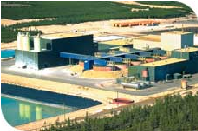
Figure 5. Key lake mill processes ore from McArthur River mine. Tailings are deposited in the Deilmann open pit. Source: Cameco Corporation.
