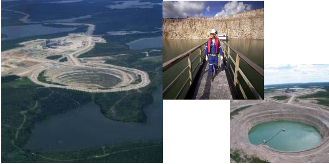
Figure 9. Left – overview of McClean (JEB) mill with ore stockpiles to the left, JEB Tailings Management Facility (TMF) in the foreground and the camp to the right; Centre and right – JEB TMF with tailings covered by water.
