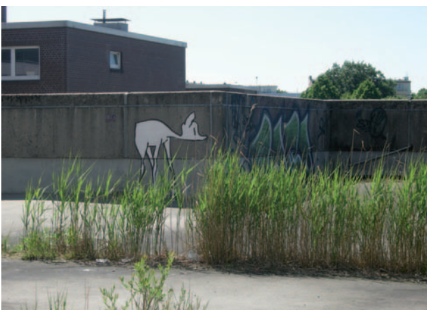
Parkdeck Frappant, Altona
