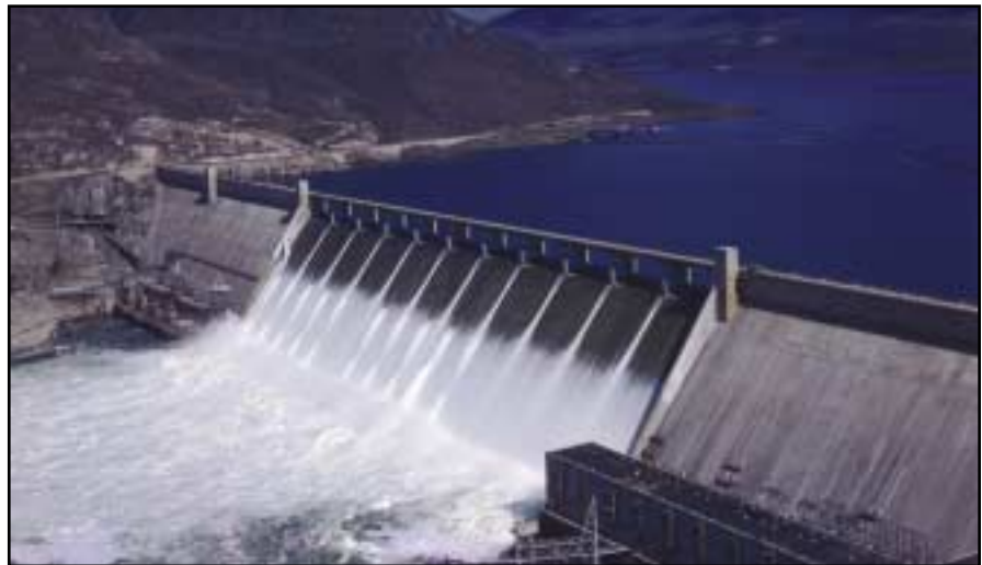
This dam's hydroelectric power plant is the largest producer of electricity in the United States, and the third largest in the world.
