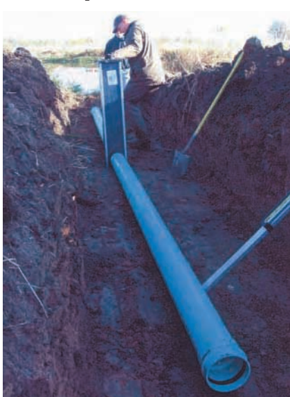
Control structure installation.
