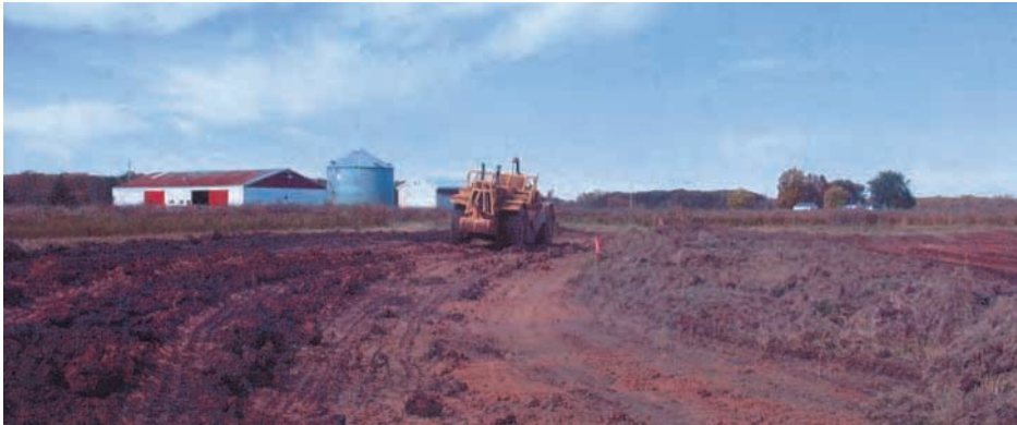
Construction started on November 18, 2005.
