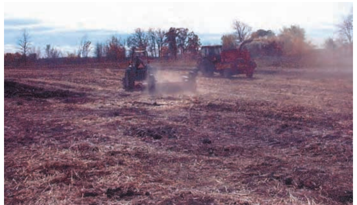
Mulching and cultipacking the berm.
