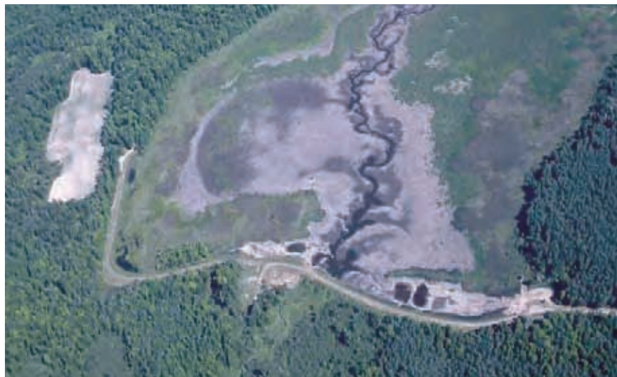
Shoulder Creek Impoundment in drawdown for repairs.
