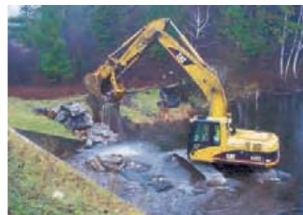
Removing concrete weir from Swamp Creek.
