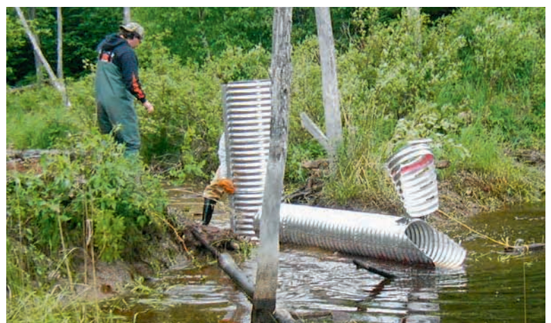
Water level control structure being installed in Eagle Bay Wetland Complex.
