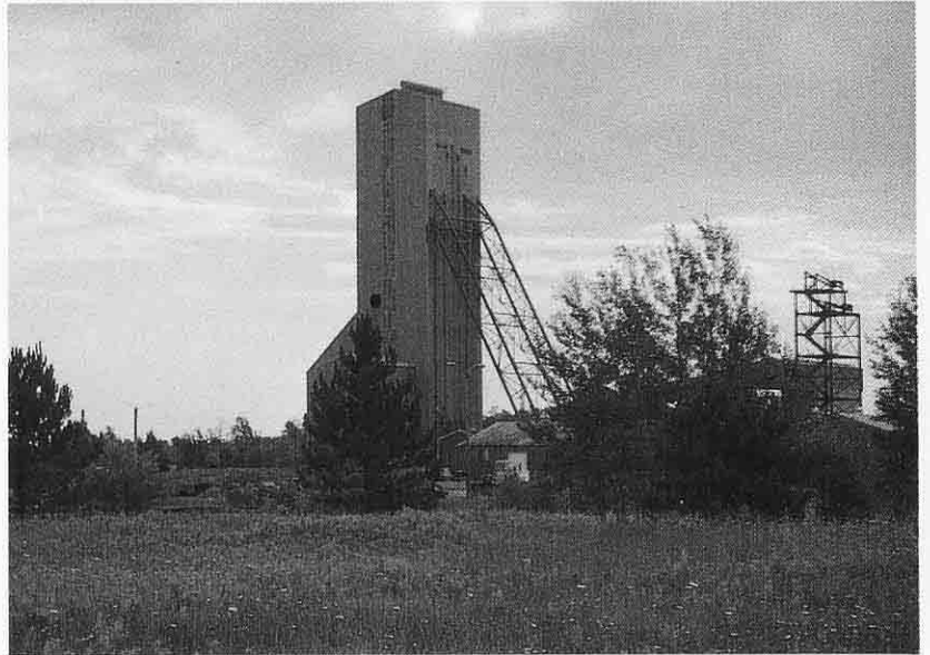
Access shaft at a mine in Michigan's Upper Peninsula.
