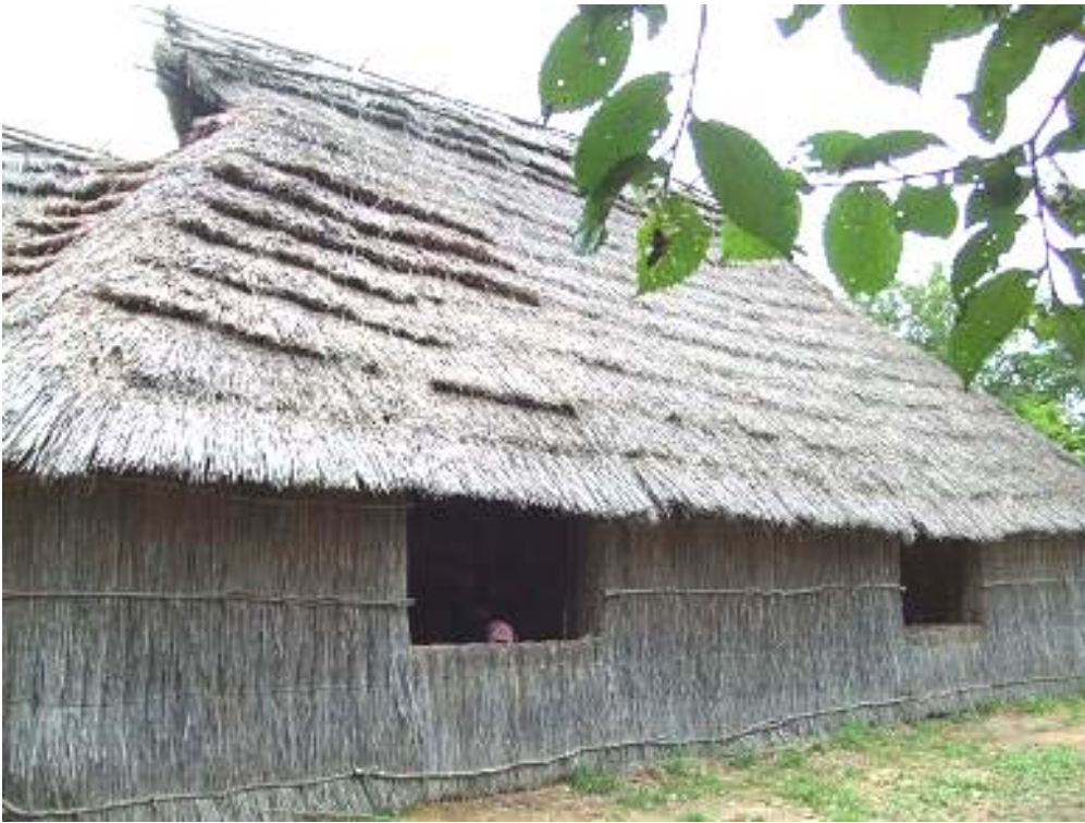
Chise (the house, in the Ainu language): The Ainu house is made out of kaya , which are thatch plants. The Ainu lived in such dwellings until about 100 years ago. These houses are still maintained for traditional ceremonies and spiritual purposes; the structure of the Ainu house follows certain rules relating to the Ainu spiritual world. There is usually a window in the east side to welcome kamuy (a spirit) from the outside to the inside of the house, which is a common belief in the Ainu culture. Inaw – sacred, peeled sticks symbolizing birds – accompany a man’s prayers to the spirit world. Photo: Kanako Uzawa
