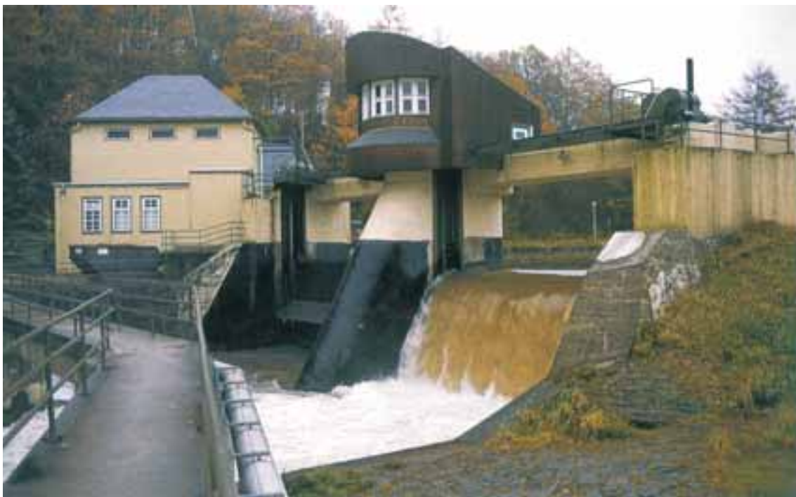
Photo 3: Dams and weirs, regardless of their height, block fish passage if not equipped with well-functioning fish passage facilities for upstream and downstream passage. The photo shows the weir of a hydropower station on a tributary to the river Rhine where Atlantic salmon once was common. (Photo: G. Marmulla).
