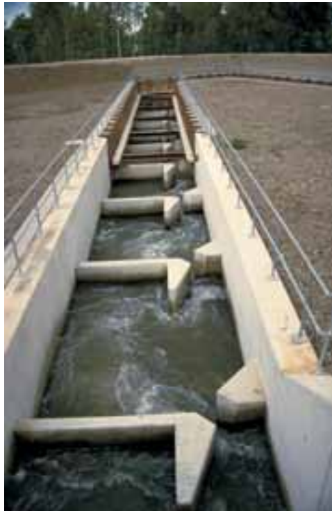
Photo 5: The vertical slot fish pass at the Iffezheim dam is an example of a recently built fish pass facility on the river Rhine. Together with the sophisticated entrance construction (i.e. several entrances to attract fish towards the pass), the 37 pools help fish to pass the 10 m high obstacle (Photo: M. Larinier).
