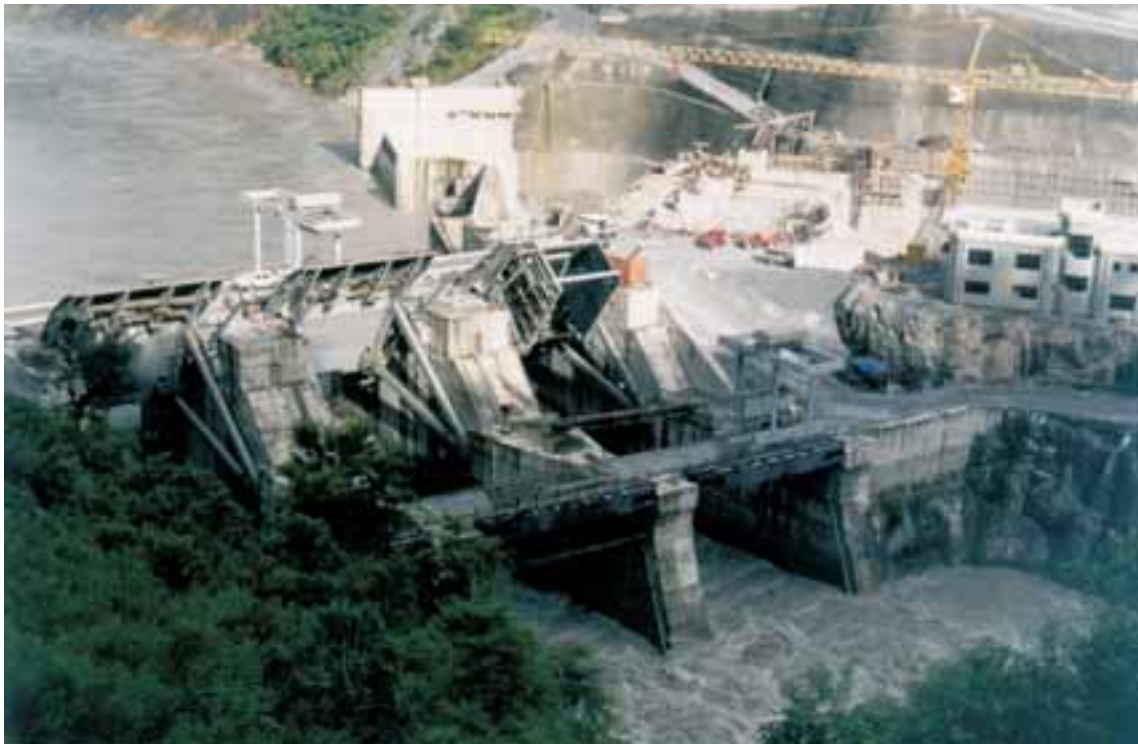
Photo 2: The dam of the Kali Gandaki “A” Hydroelectric Project in Nepal (still under construction when the photo was taken in July 2001) is a typical example of an obstacle that blocks the migratory route of fish species that are important for the river fisheries as no fish pass was constructed for upstream migration. (Photo: G. Marmulla)
