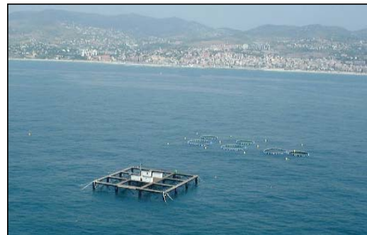
12. Platform cage, Spain, circa 2000. Uses oil field type structure fixed to sea bed for net support
