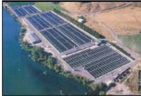
Clear Springs Trout Farm in Idaho uses concrete raceways supplied by spring water
