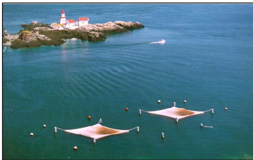
5. Ocean Spar cage circa 1990. Relies on anchor tension to hold shape. Partly submersible but has not done well in really heavy sea conditions.
