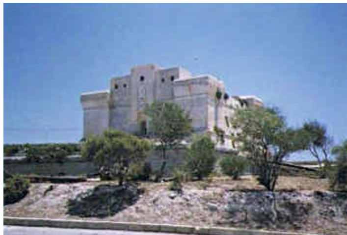
National Aquaculture Centre, Fort San Lucjan, Marsaxlokk
