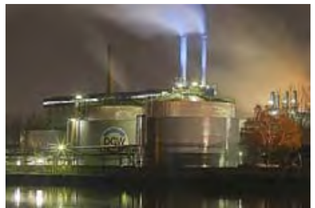
2 Stromerzeugung und Fernwärme aus Steinkohle Electric power and district heating by process heat from carbon black production.
