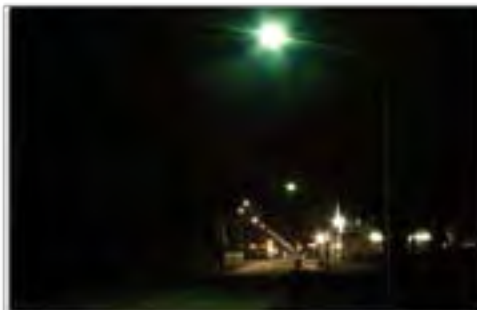
The old equipment, fitted with two 125W mercury-vapor, high-pressure discharge lamps, can be seen in the foreground.
