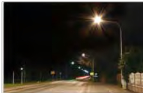
The modernized equipment, viewed from the opposite direction, with modern Kaffir-line luminaires fitted with CosmoPolis 60W.
