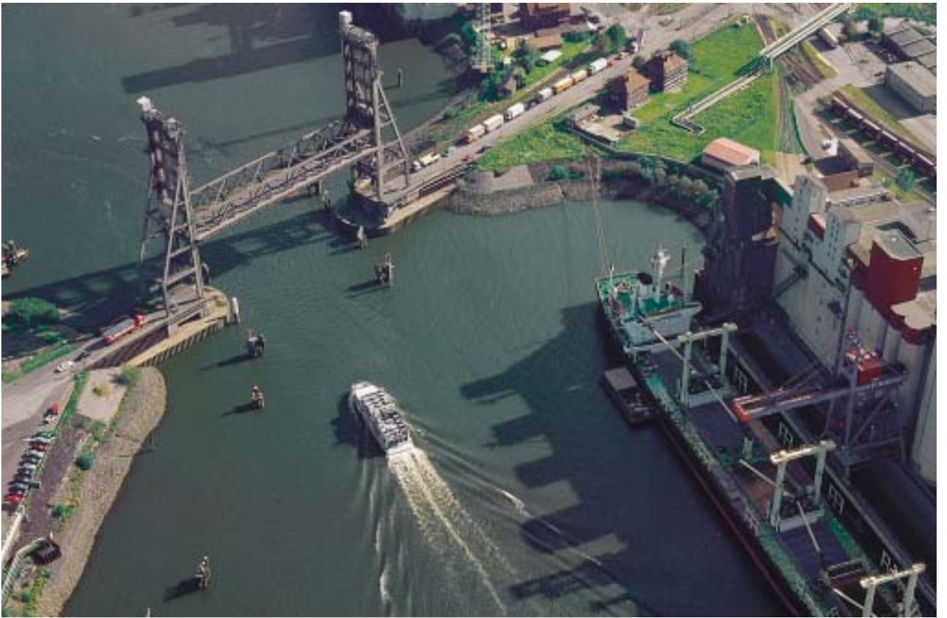
Rethehubbrücke / Lift bridge Rethehubbrücke
