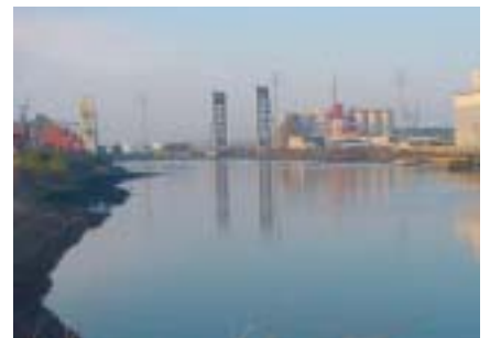
Rethehubbrücke / Lift bridge Rethehubbrücke
