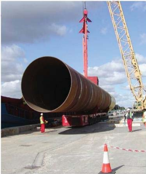
Abb. 7: Monopile (E.ON-Offshore-Project Scroby Sands)
